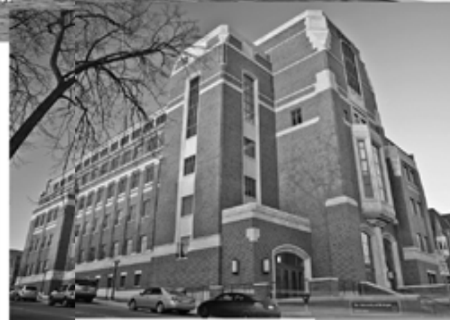
JOAN AND SANFORD WEILL HALL, GERALD R. FORD SCHOOL OF PUBLIC POLICY The $32 million, 85,000-square foot building opened its doors in August 2006. It is positioned at the corner of State and Hill Streets as a symbolic gateway to Central Campus.
